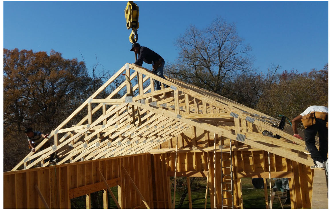
Roof for the addition
