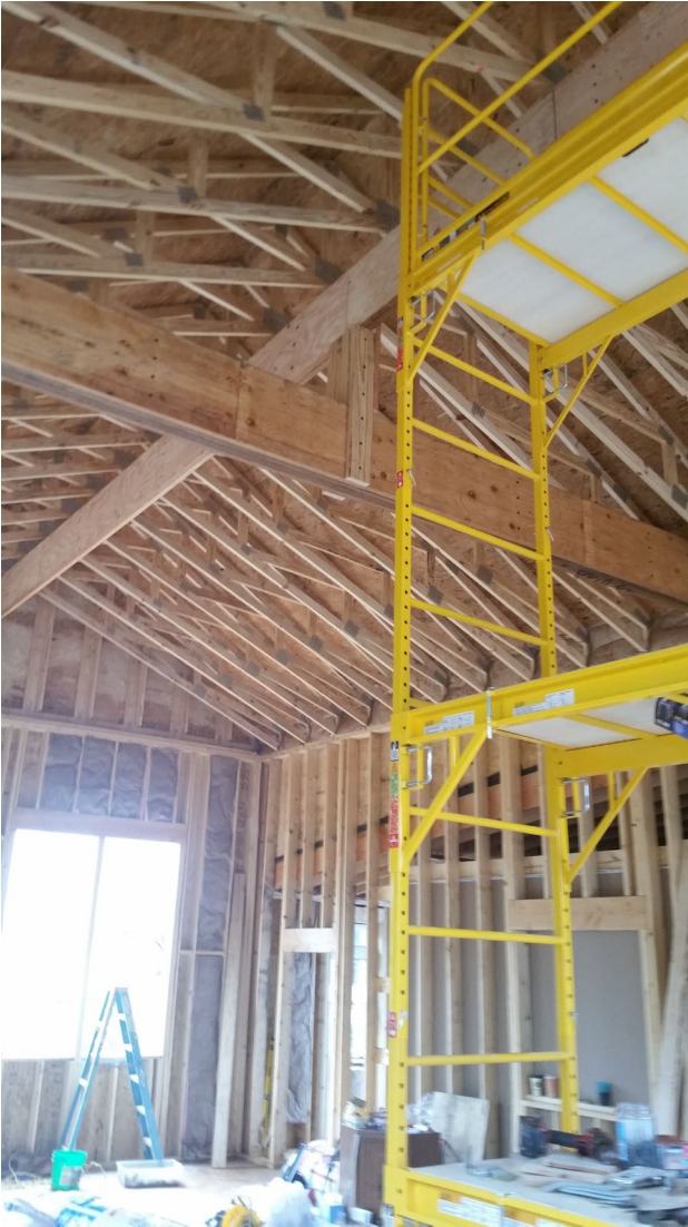
Large beam to support Aerial Room
