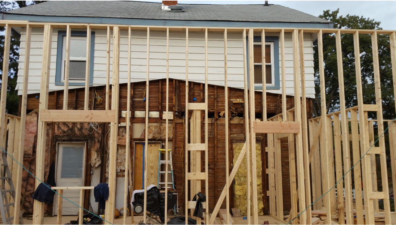
Framing for the addition
